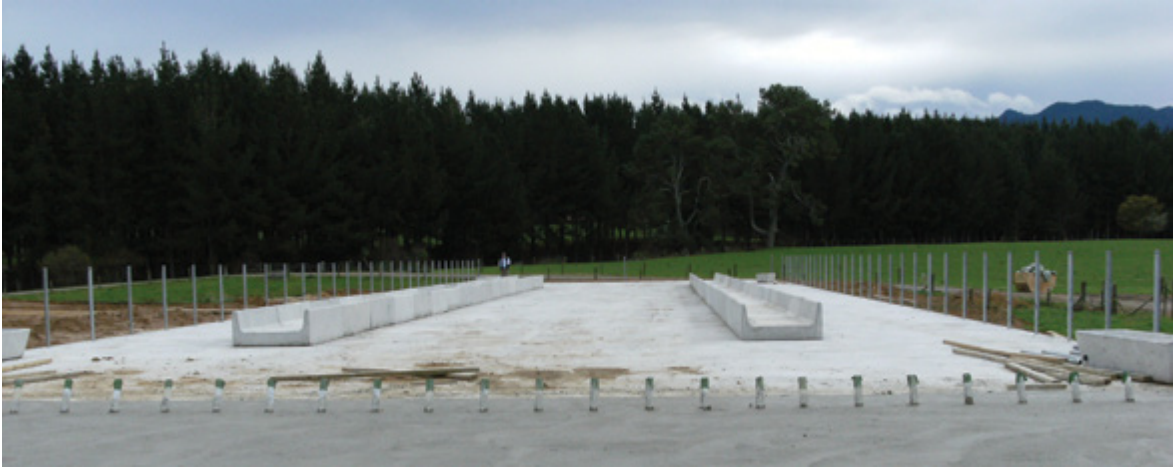
Feed pad under construction
