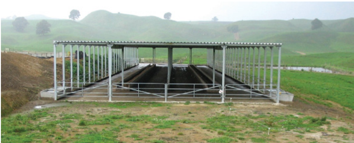
Covered feed pad
