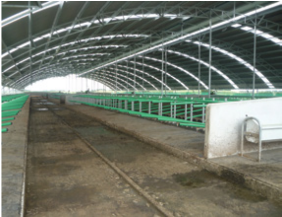
Covered feed pad
