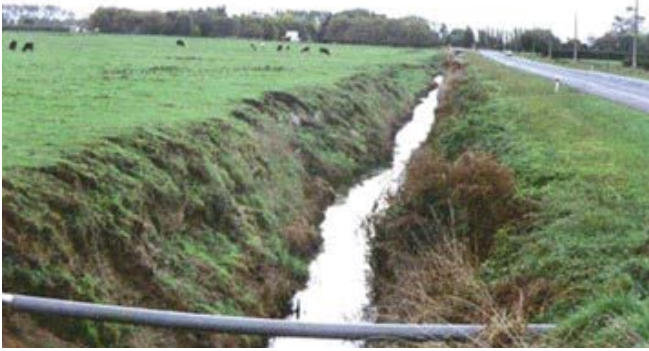
Drain bank erosion caused by stock.
