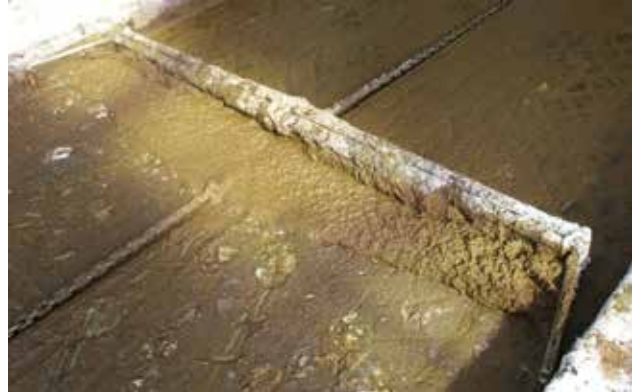
Ensure the scraper runs frequently enough to keep the volume of scraped slurry from overflowing onto the beds.
