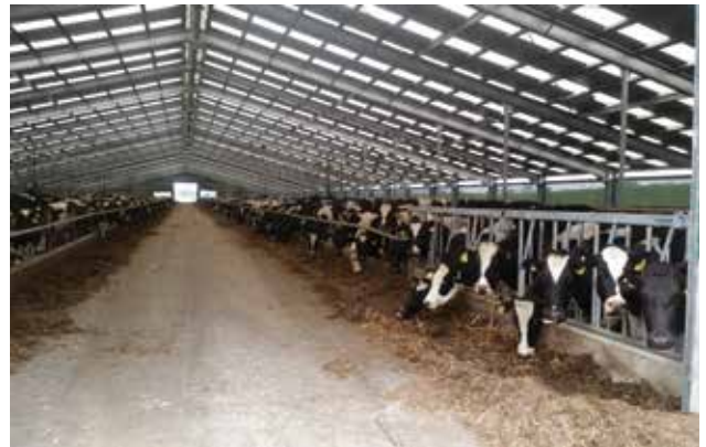
It is possible to install a few locking yokes at the end of the feed face to provide a cow handling area. Alternatively consider including a vet race in the building design.
