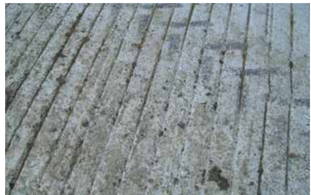
Textured concrete gives more traction without slipping
