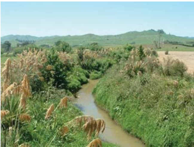
Streambank planting with low growing native plants. Using low growing plants on steep banks is important for stability and increases flow by supporting a V-profile.
