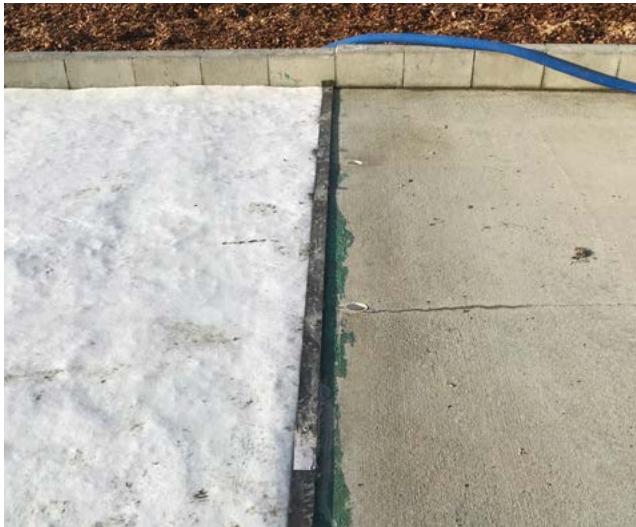
Flood wash risers imbedded in the concrete. Water flows from right to left.
