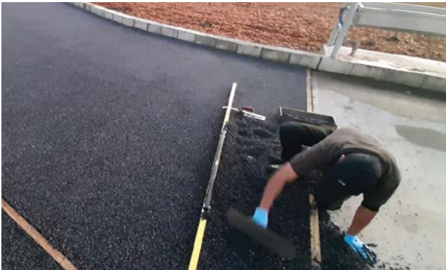
Experimental pour-in-place rubber surface prior to adhesion of a geotextile top surface.
