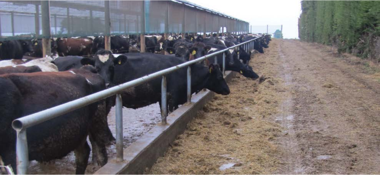
Consider wider concrete feed tables (1.2 - 1.5 metres) and durable machinery tracks to reduce feed wastage and pugging. See feed barrier (section 5, page 34) for the best design.
