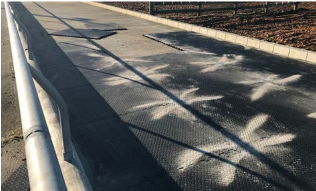
Interlocking rubber matting on concrete.
