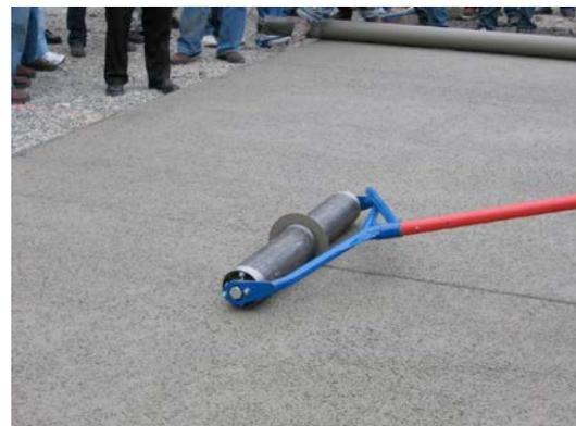
**Figure 18:** Jointing tool or T section
