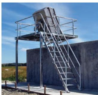
*Slope screen with platform and safety railing, access ladder at rear*
