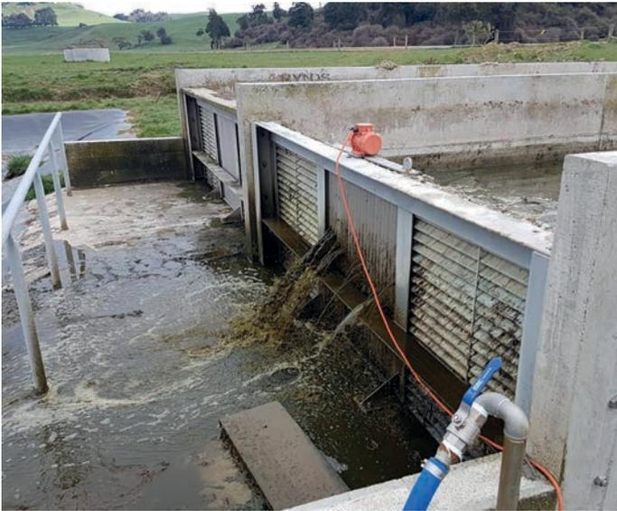
*Weeping wall (PVC outer panels, vibrating centre panel)*
