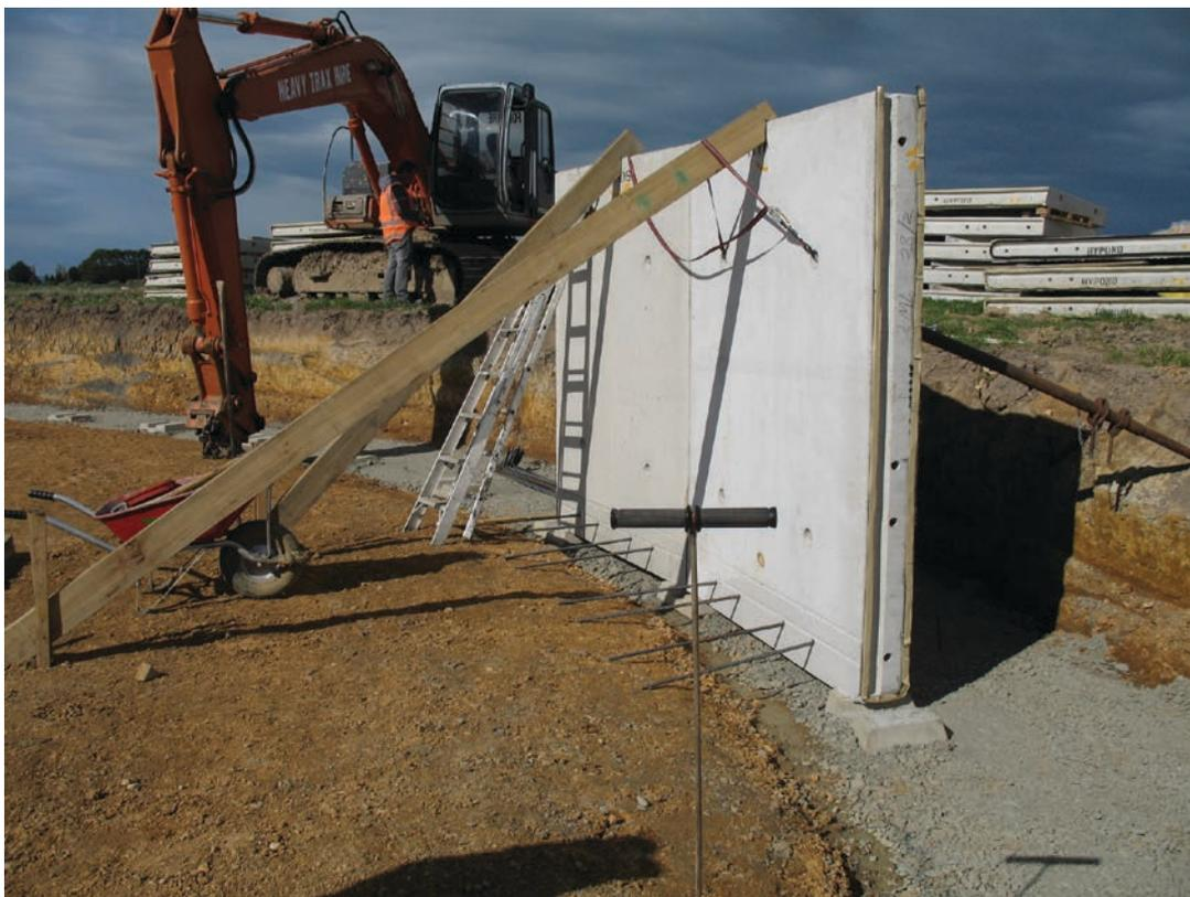
*Storage tank, precast reinforced concrete panel construction*
