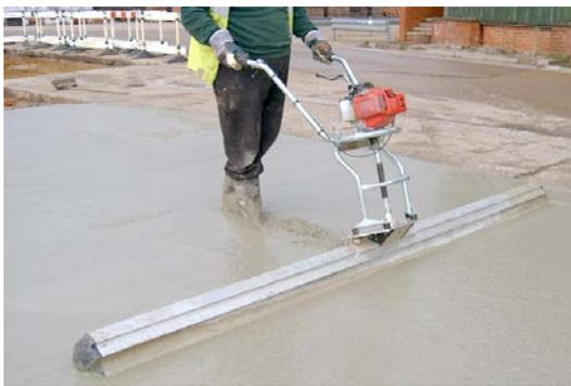
Figure 11: Lightweight vibrating screed
