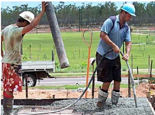
Figure 12: Immersion poker vibration
